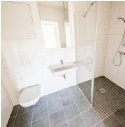
The wet cell is prefabricated and inserted into the module in the building factory.
